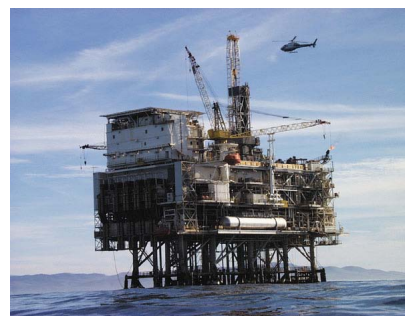
Figure 1. Oil and gas offshore platform.
