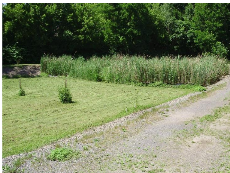
Fig. 7. Subterranean Flow Constructed Wetland Cell 1 [31]
